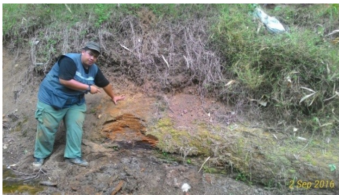
Figure 9. Condition of Weathered Outcrop in the Northern Part area
